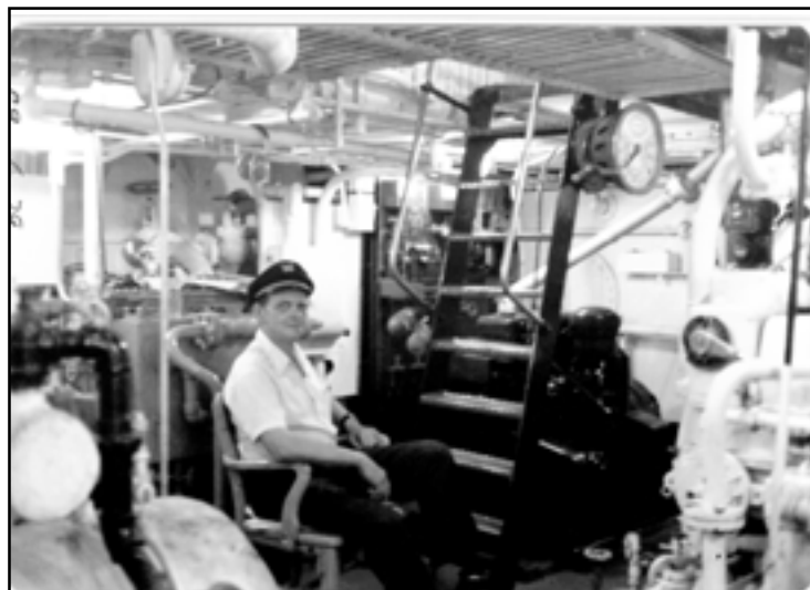
The Engine Room of the Amherst Islander, c.1979 with Engineer Tom Miller SM Photo
