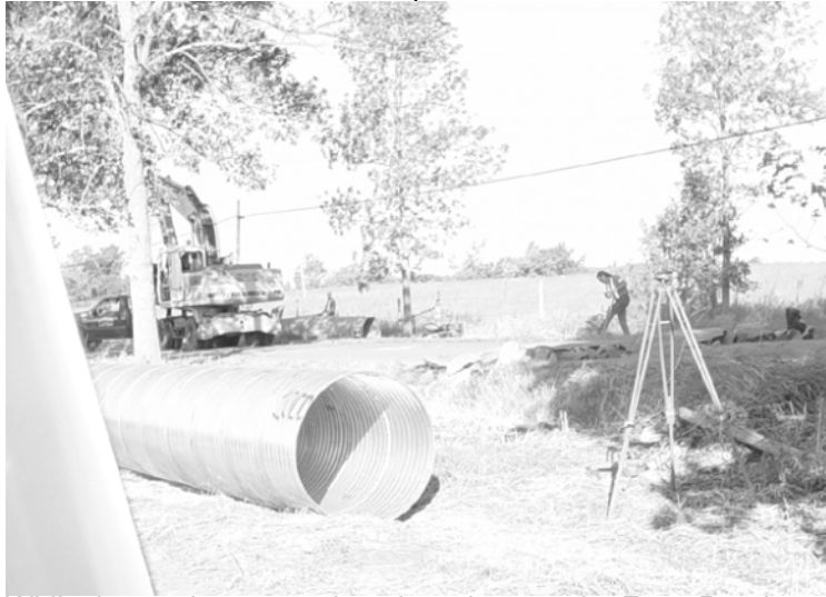
While the roads crew replaced a culvert on the Front Road near Vincent Eves' farm in September 2002, traffic profited from a scenic detour through a nearby cornfield. TR
