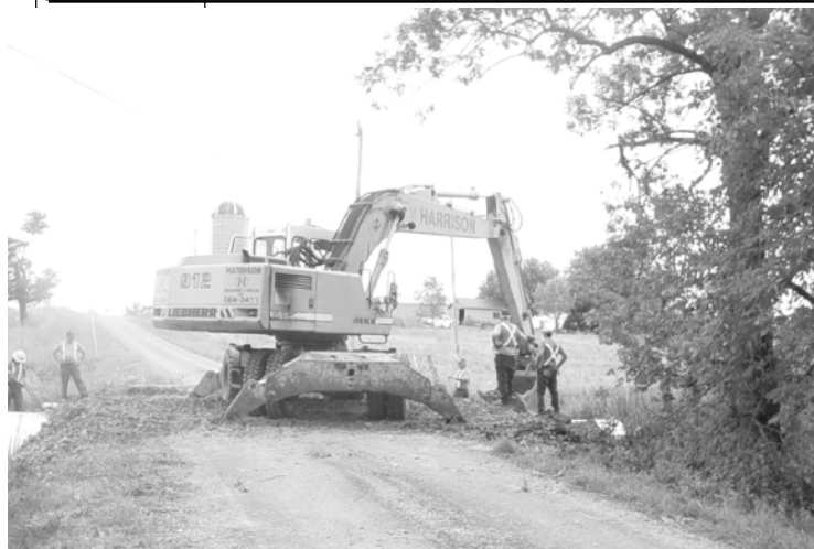
The AI Roads Crew replaces the bridge on Art McGinn's Road with two large steel culverts, September 2002 TR
