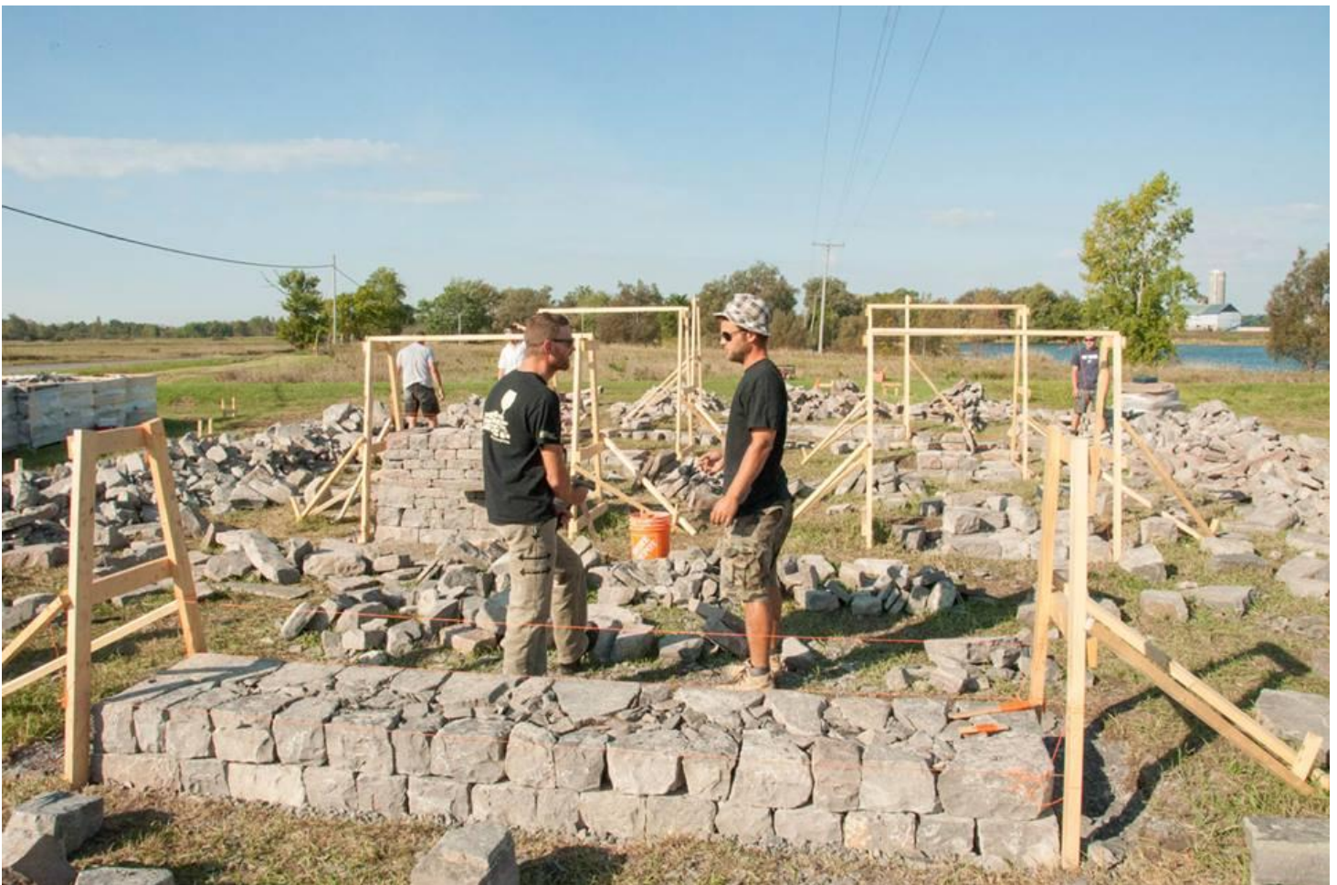
Kenneth Curran and John Bland starting to build within batter frames
