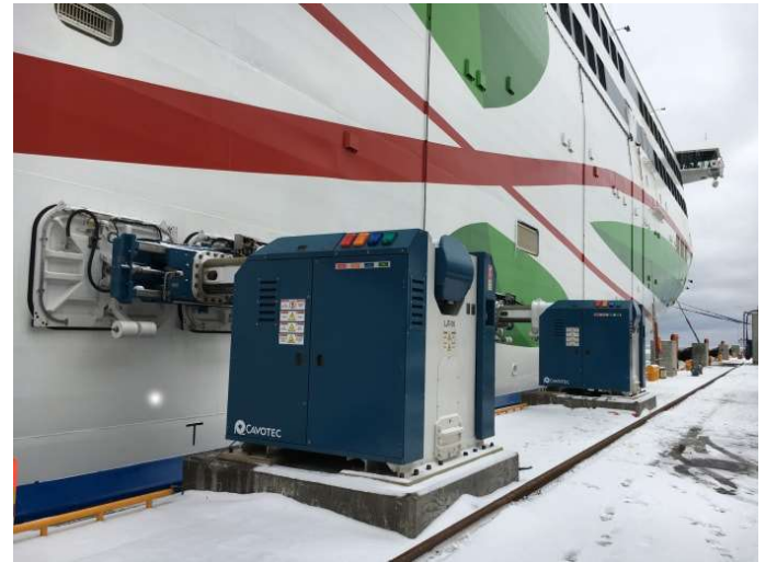
The MoorMaster system eliminates the need for rope-based mooring. Vacuums hold the ferry.
